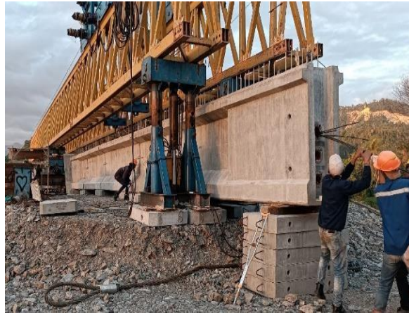
Gambar 4. Proses install PC strand
