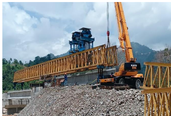
Gambar 3. Proses levelling girder
