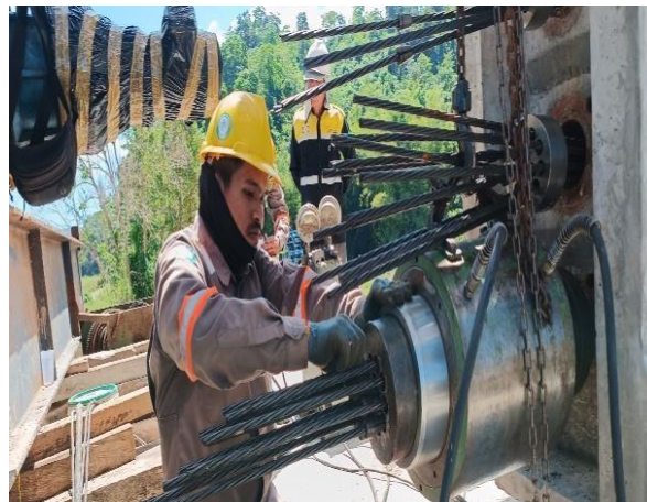
Gambar 5. Proses install PC strand
